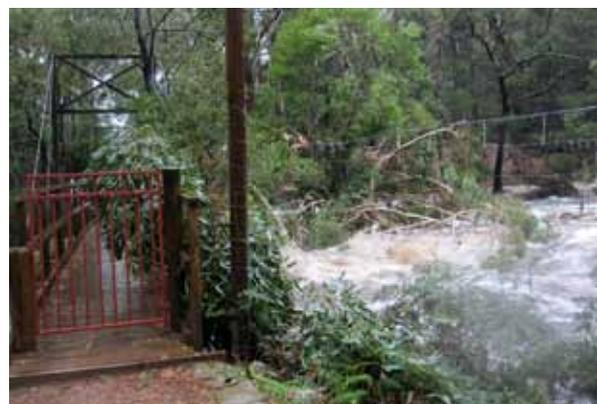
Trees coming down the creek bent the bridge, and it needs replacing rather than repairing. Photo by Margo Sietsma
